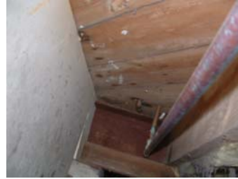
Photo 8 – No Insulation
