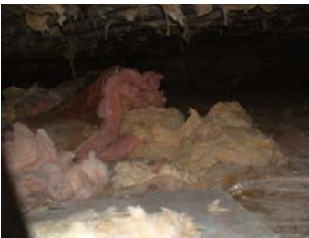
Photo 22 – Debris/Single Layer Battis
