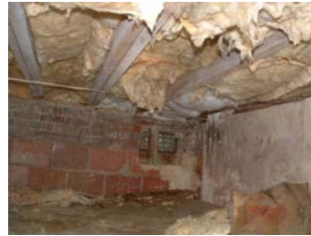
Photo 28 – Moisture/Single Layer Batts
