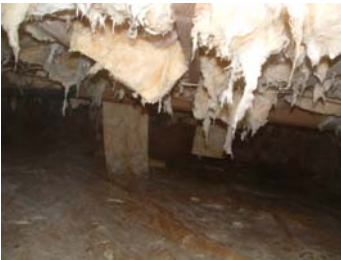
Photo 55 – No Wire Lacing
