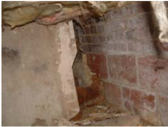
Photo 24 – Incomplete Firewall
