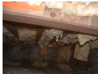
Photo 47 – No Wire Lacing/Single Batts
