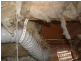
Photo 44 – Missing Insulation
