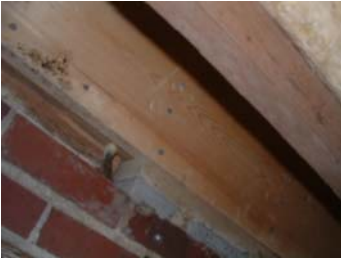
Photo 54 – Missing Insulation
