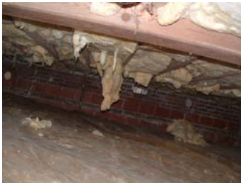
Photo 32 – No Wire Lacing/Single Layer Batts
