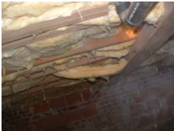
Photo 25 – Incomplete Wire Lacing
